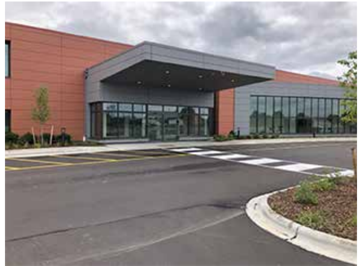
Mary Beulow, photos Dr Daniel Hale Williams Resource Center's west entrance, facing Center Street
